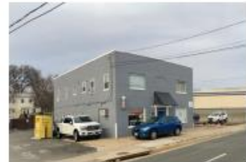
Existing condition at the Moore's Barber Shop building on the north side of Langston Boulevard
